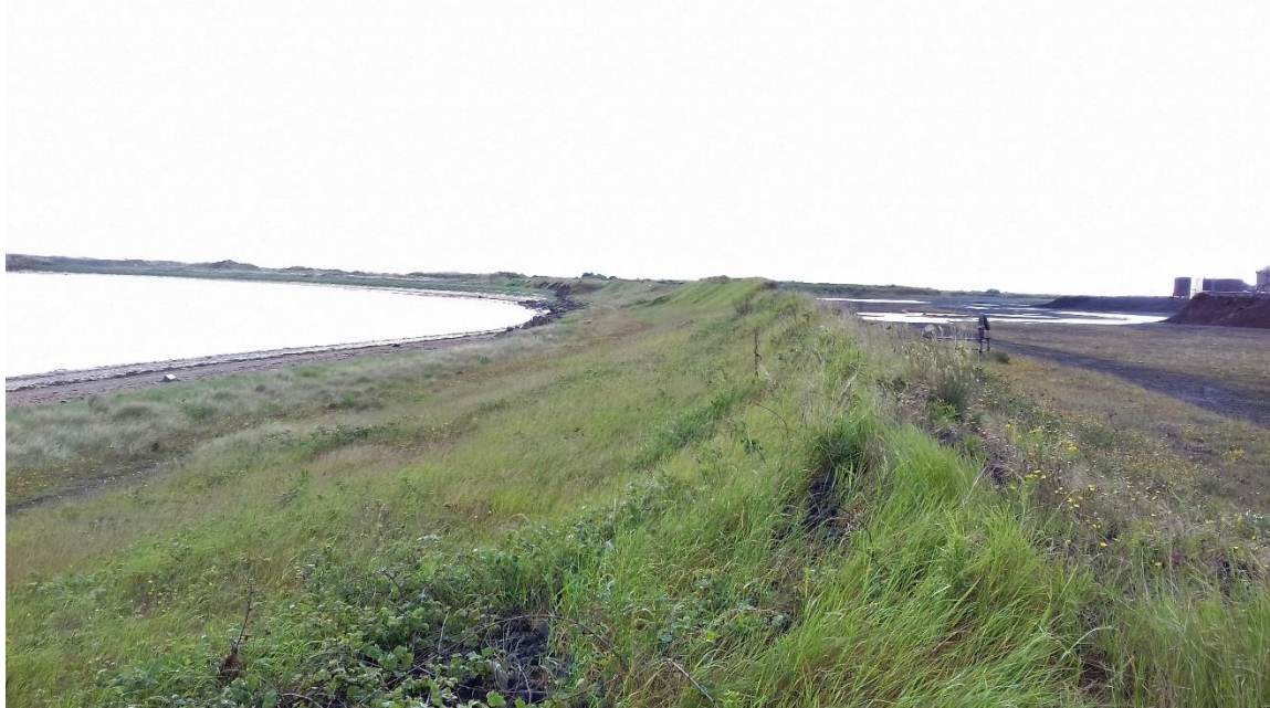
Photo 2: The bund to the north and north east of the Application Site with semi-improved grassland separating the site from the coastal sand dune system.
